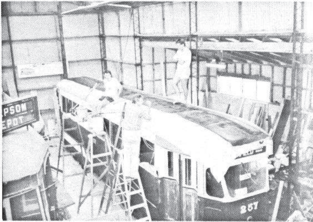
Laying butyl rubber on the roof of Fiducia 257 at MOTAT. Photograph: Ian Stewart.
